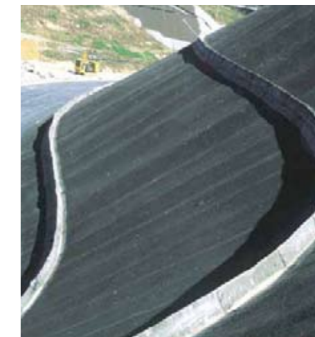
Rain water divert channels stuck onto the barrier. These channels prevent excessive rainwater entering the cell. They can be removed or simply left in place without fear of damaging the barrier
